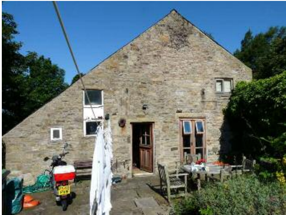
Fig.3: the altered east gable-end; all openings date from the 1988 conversion
