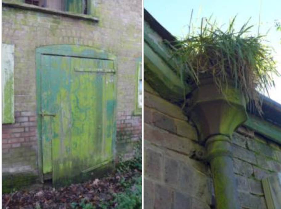
Figures 4.13 and 4.14: Typical Door and Remaining Rainwater Good
