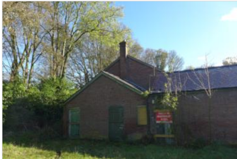
Figure 4.10: Western Elevation of Combination Barn
