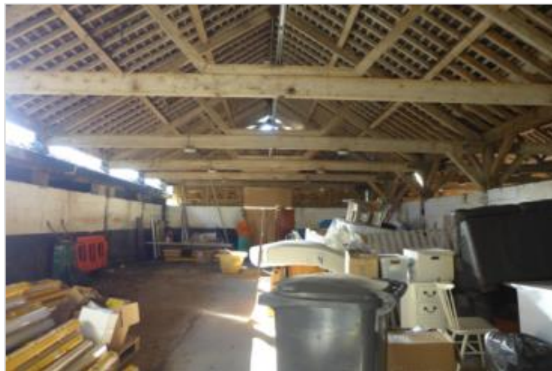
Figure 4.24: Interior of Covered Yard
