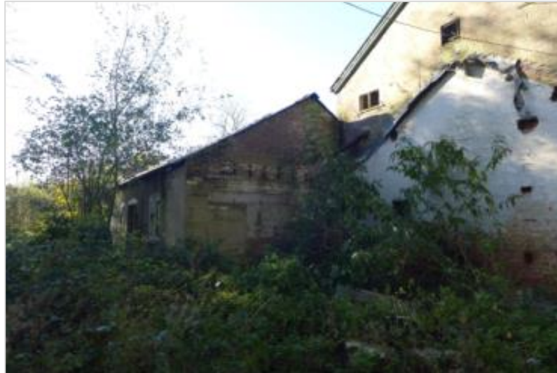
Figure 4.11: Scar on Eastern Elevation of Combination Barn
