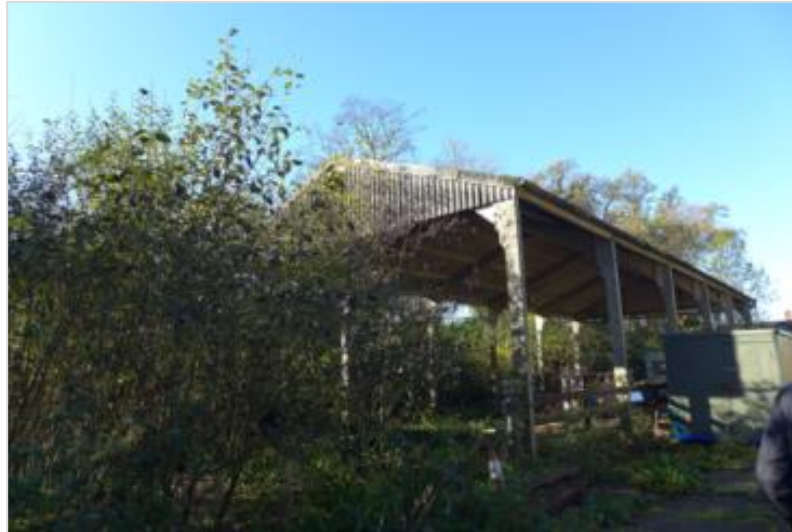
Figure 4.26: Late 20 th Century Ancillary Building
